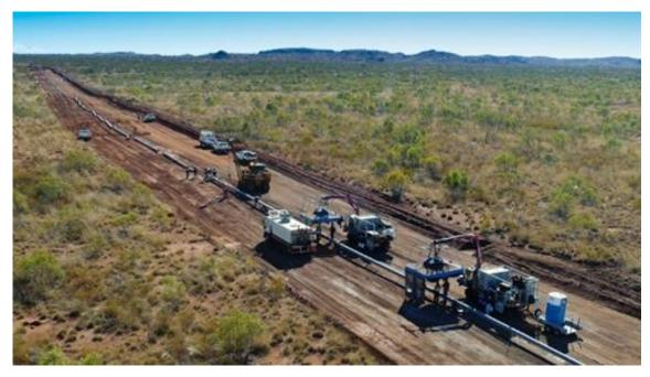
Figure 11: Welding crew operating on the pipeline right of way (Spiecapag Australia)
