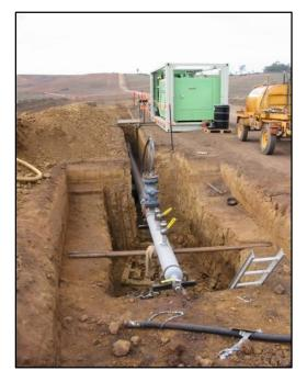
Figure 25: Hydrostatic testing a section of pipeline. (Ecos Consulting)
