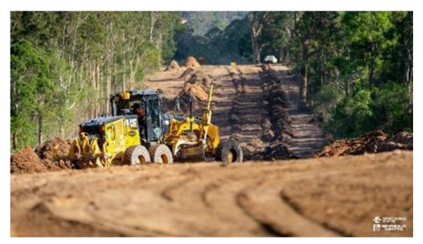
Figure 14: Grader operating during clear and grade (Spiecapag Australia)
