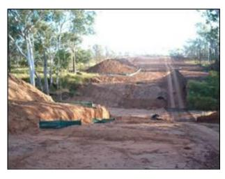
*Figure 8: Erosion controls (berms and sediment fences) at a watercourse crossing. (W. Mathieson)*
