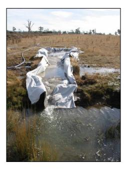
Figure 9: Erosion controls at a trench de-watering site. (Ecos Consulting)
