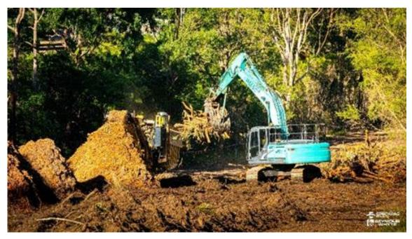
Figure 15: Vegetation clearing and stockpiling (Spiecapag Australia)
