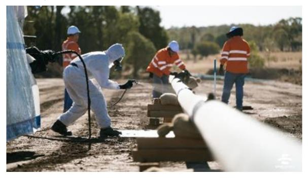
Figure 16: Mainline coating being undertaken (Spiecapag Australia)
