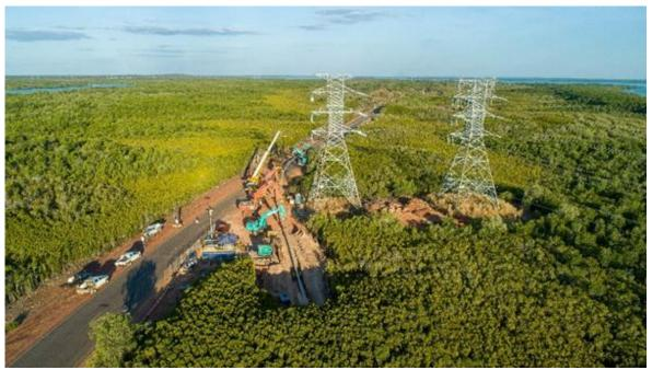
Figure 22: HDD Exit Side Pipe Pull Back operation (Spiecapag Australia)
