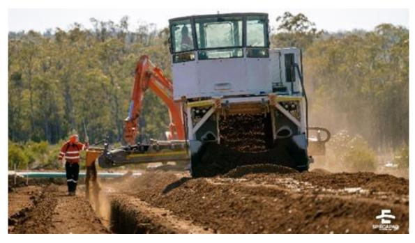
Figure 24: Backfill padding (Spiecapag Australia)
