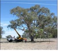
Figure 16 Trimming overhanging vegetation on a pipeline corridor as part of clearing activities (Ecos Consulting)
