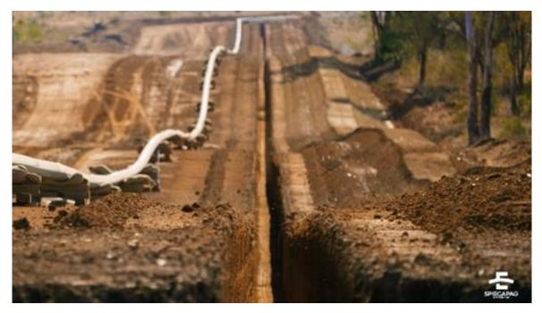
Figure 17: Welded pipeline ready to be lowered into the open trench (Spiecapag Australia)
