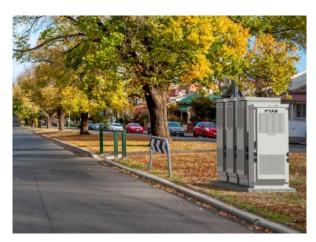
**Figure 1:** A pad mounted battery storage facility, Source: Yarra Energy Foundation, Sydney
