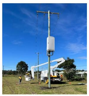
**Figure 4:** A pole mounted battery storage facility, Source: Energy Queensland
