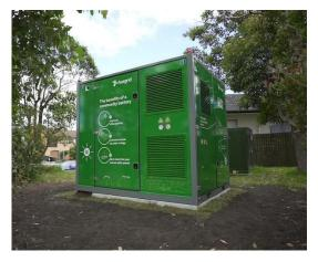
**Figure 2:** A pad mounted battery storage facility, Source: Ausgrid, Sydney
