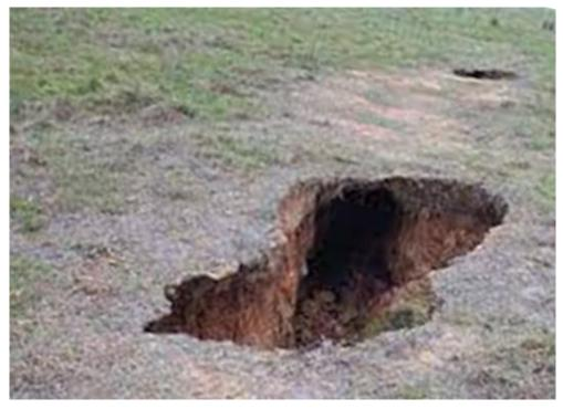
Figure 5 - Example of tunnel erosion or sinkhole over pipeline
