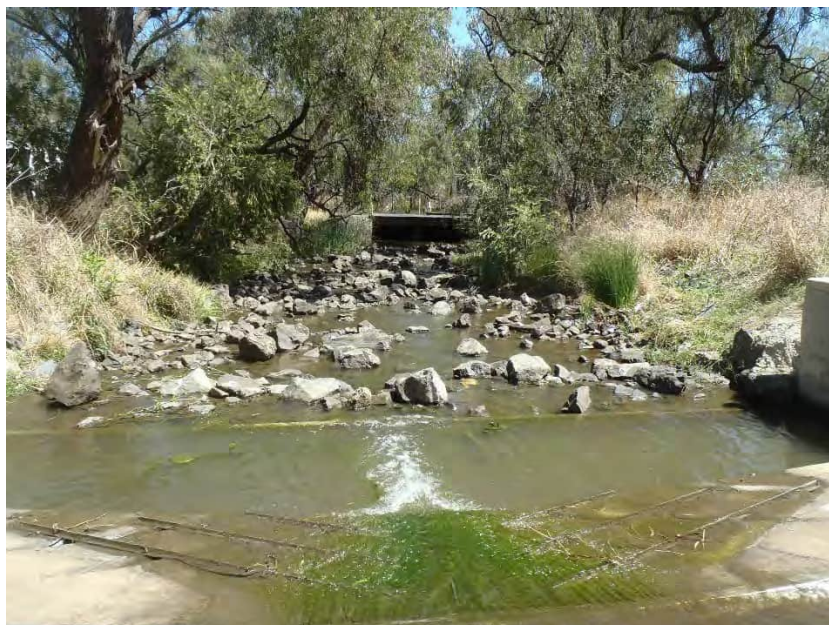
Picture 3-6 Typical rock-ramp fishway structure
